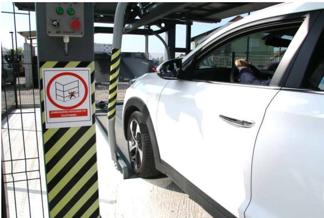
Figure 14: Correct positioning of the wheels during vehicle entry
